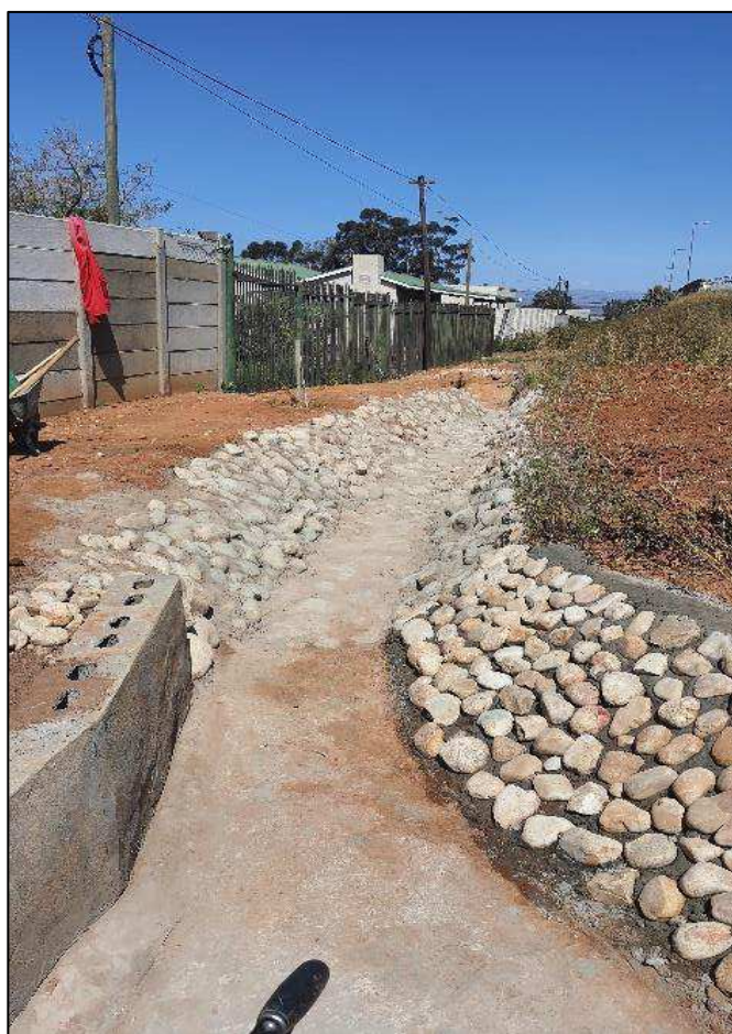
STONE PITCHING AT THE OPEN STORMWATER CHANNEL ADJACENT TO BREUSING STREET
