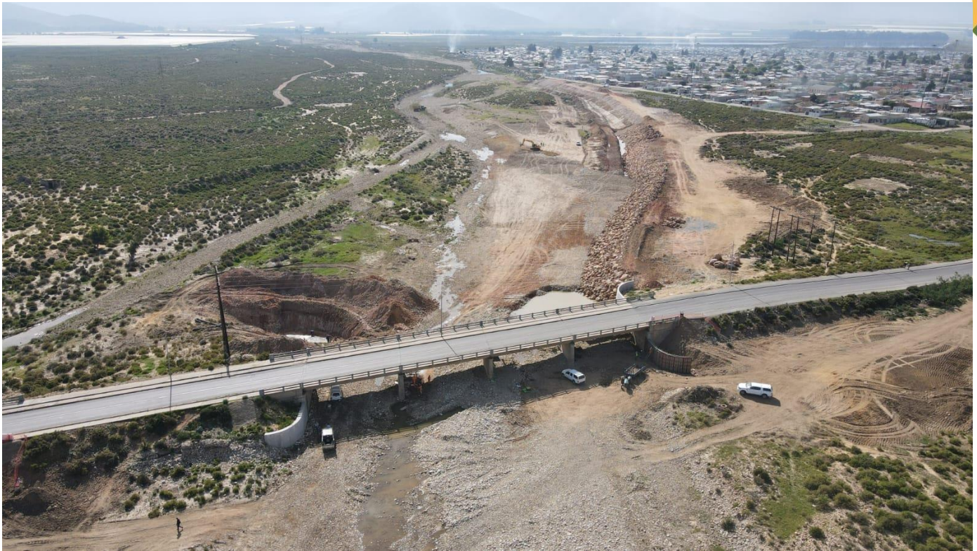
CONSTRUCTION OF HEADWALLS UPSTREAM AND DOWNSTREAM OF ACCESS BRIDGE TO ZWELETHEMBA
