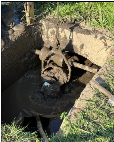
SILTATION AND DEBRIS REMOVED FROM THE ROBERTNSON ROAD UNDERGROUND STORMWATER CONDUIT
