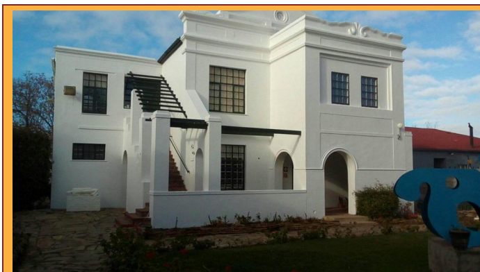
Maintenance at Jean Welz Gallery
