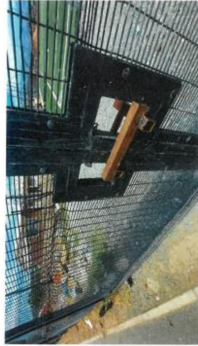
RSEP in Avian Park: gates welded shut, locked away from the community.
