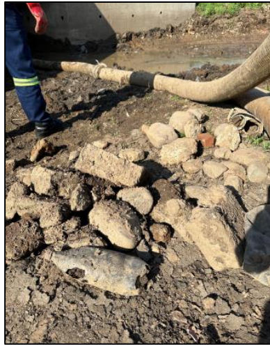
SILTATION AND DEBRIS REMOVED FROM THE ROBERTNSON ROAD UNDERGROUND STORMWATER CONDUIT
