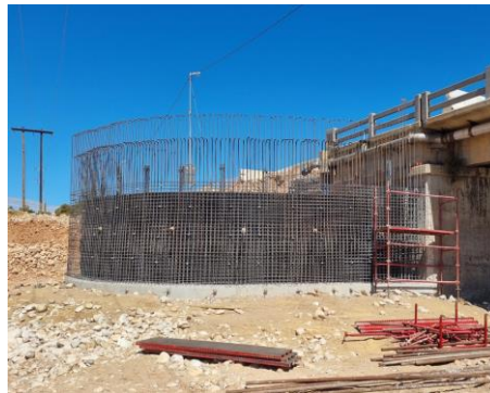
TYPICAL DETAIL OF HEADWALL AT ACCESS BRIDGE TO ZWELETHEMBA
